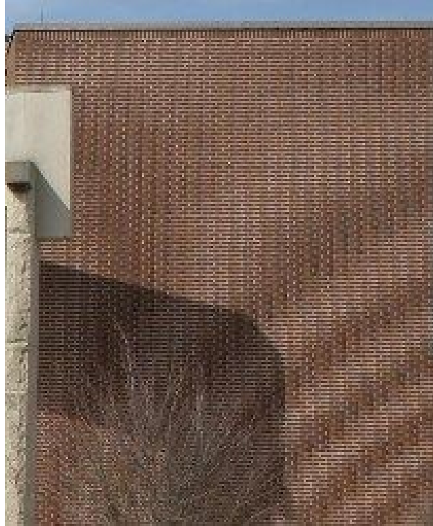
Figure 3 Radial moiré pattern is created by downsampling the image of a brick pattern.
