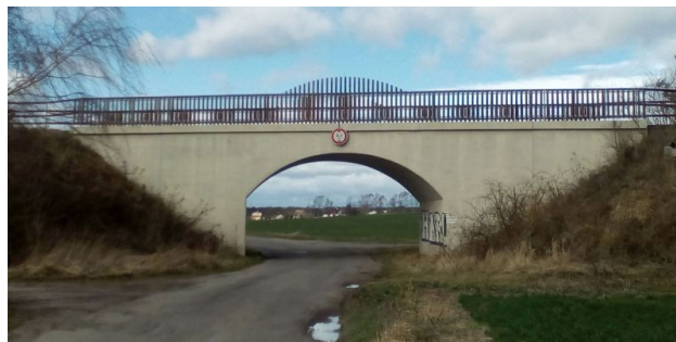
Figure 1 Example of moiré pattern created by two layers of overpass fencing.
